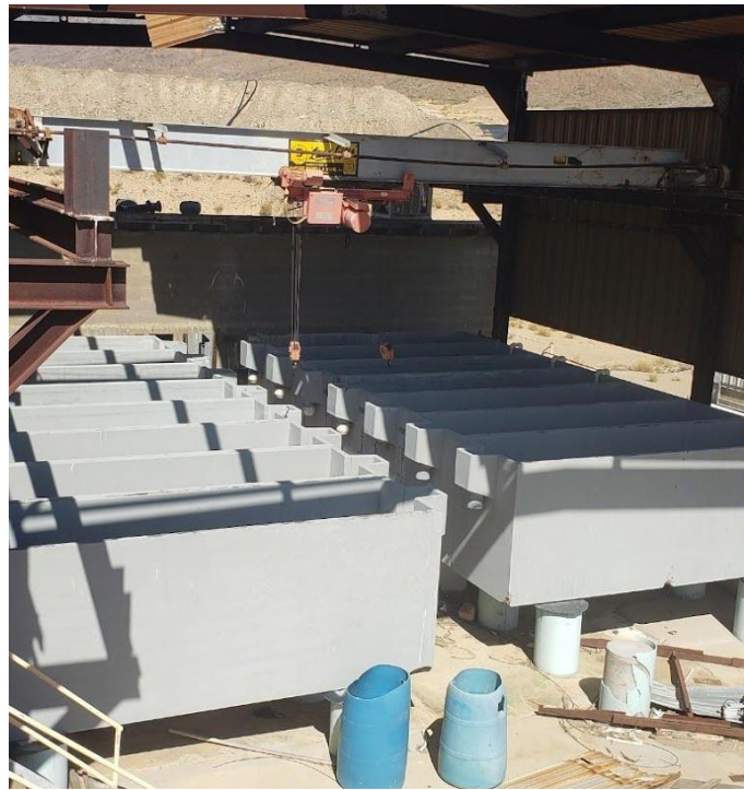
Figure 3.4: Abandoned Electrowinning Equipment (photo credit - Sydney Adamonis)
